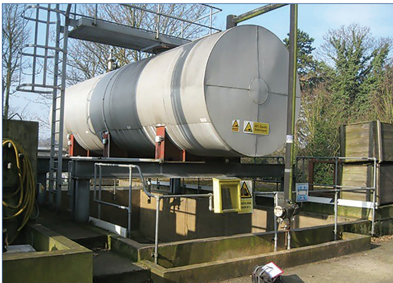
Figure 6.4 Example of installation vulnerable to jetting of fuels over the bund wall (courtesy CH2M Hill, with permission from the Environment Agency)
