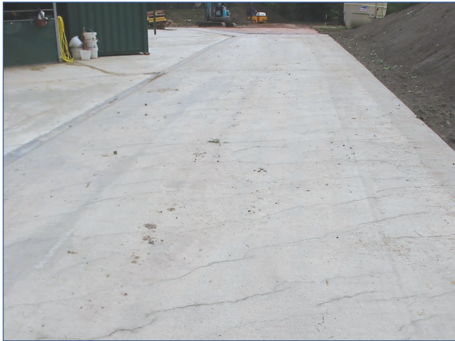
Figure 7.6 Plastic shrinkage cracks (courtesy Concrete Society)
