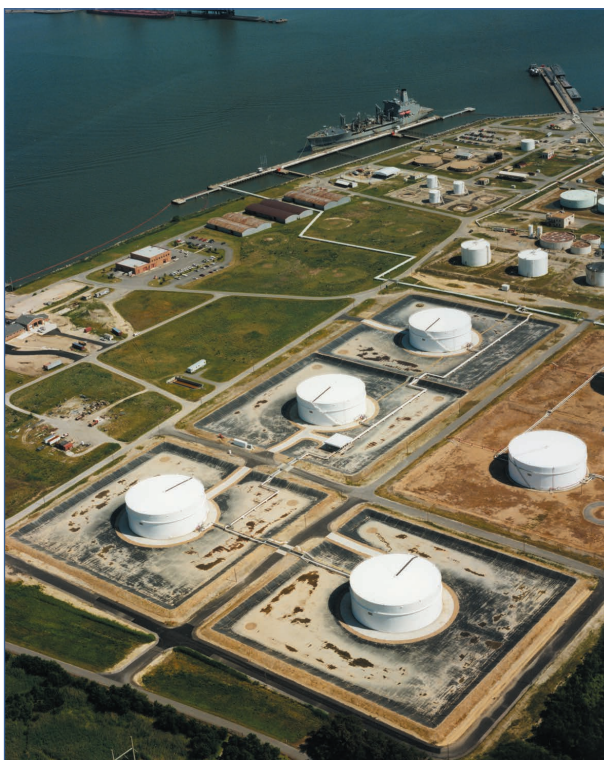
Figure 6.3 A compartmentalised bund (courtesy Seaman Corporation)
