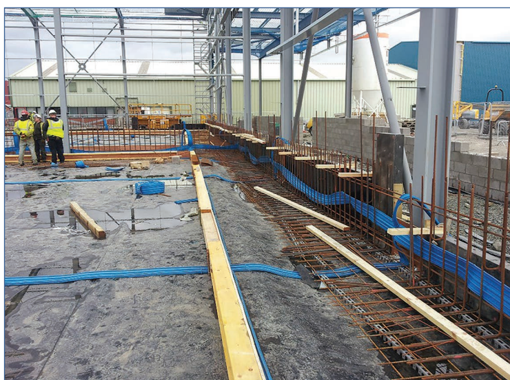
Figure 7.5 Waterstop tied into reinforcement cage at the kicker and rear face waterstops at the planned slab joints (courtesy H W Coates Ltd)
