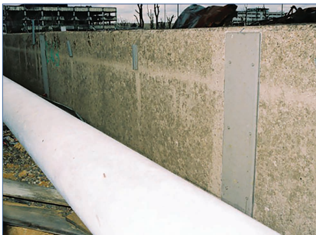
Figure 5.11 A plated joint (courtesy CH2M Hill, with permission from the Environment Agency)
